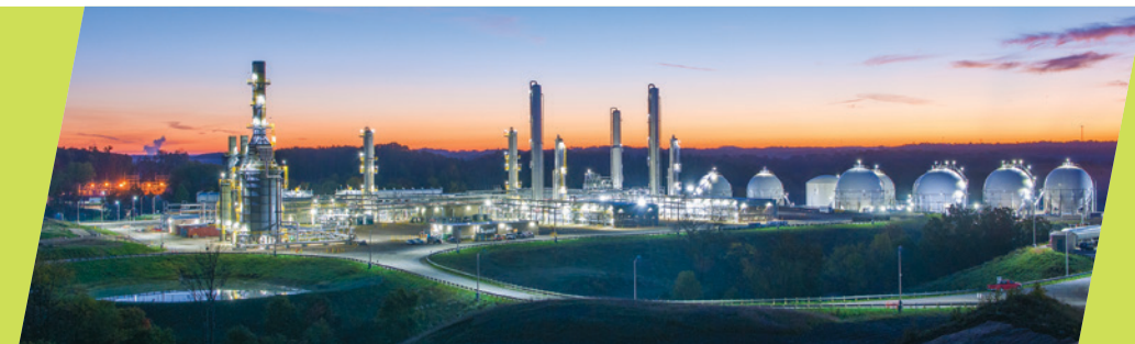
MarkWest Energy Partners, Hopedale facility
