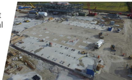
Oregon Clean Energy Center under construction
